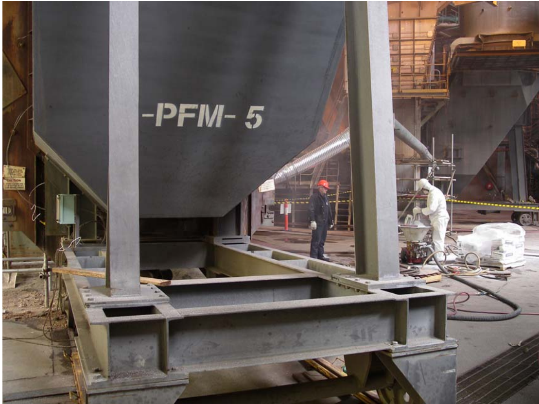
November 2006: Thermbond gunning repair operation at Loy Yang Power Mill door
