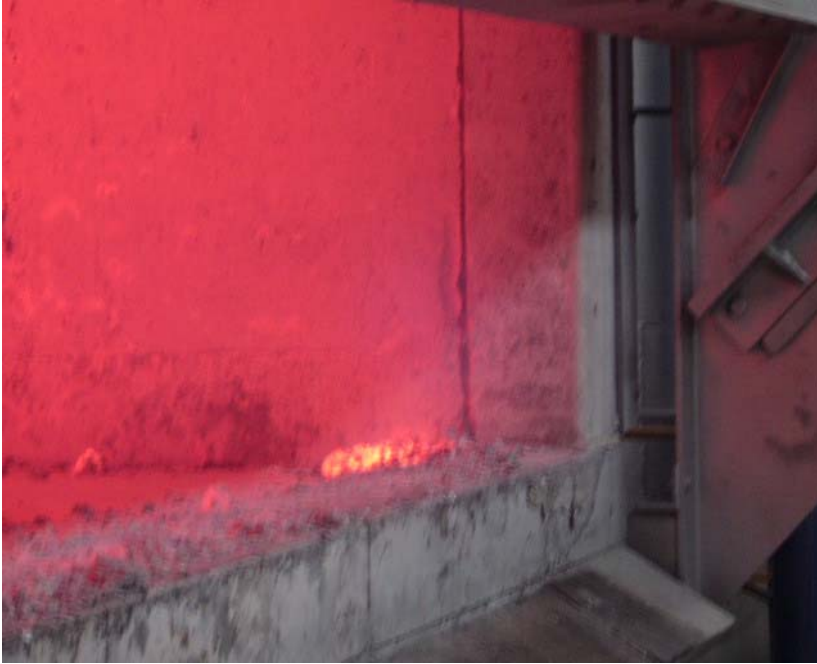
Photo 1. shows the door jamb block construction
