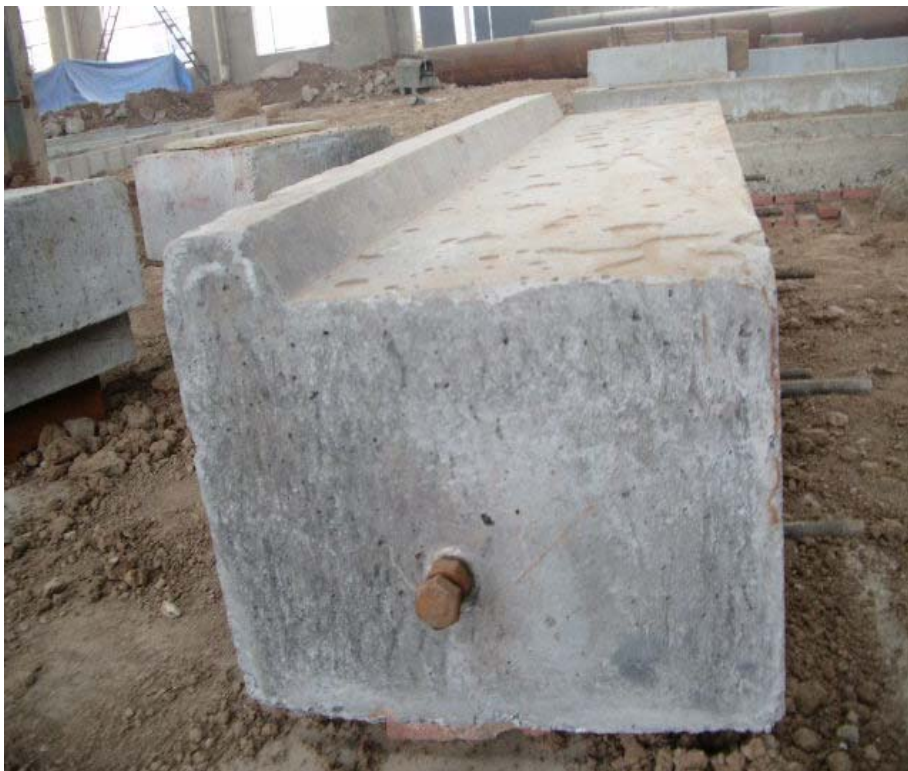
Refractech Pre-cast block design for door lintel and jamb
